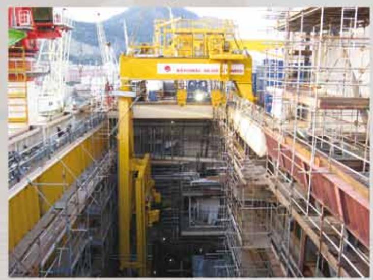
Installation of "BOP Over Head Crane" on SAIPEM "SCARABEO 8" drilling rig (Fincantieri Palermo shipyard)
