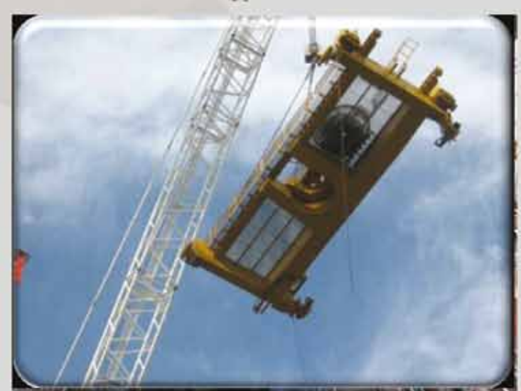
Installation of "Baseplate Trolley" on SAIPEM "SCARABEO 8" drilling rig (Fincantieri Palermo shipyard)
